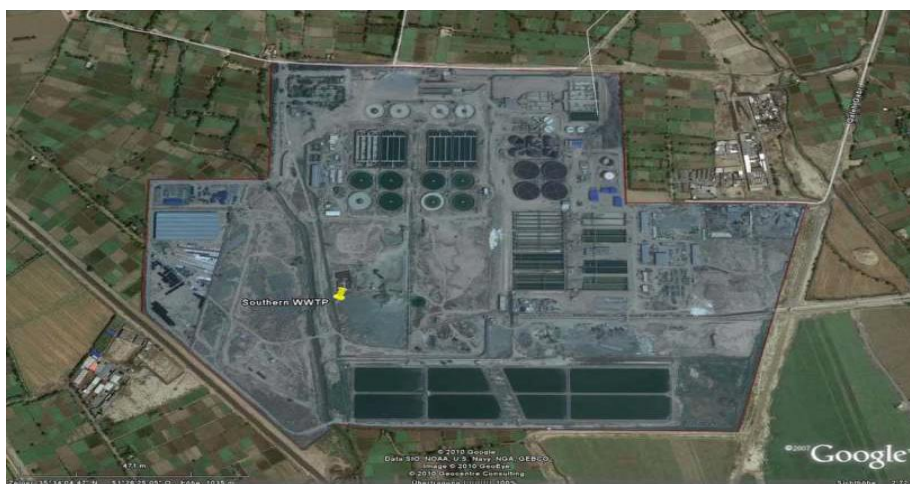
Figure 1: Tehran South Wastewater Treatment Plant facilities.
