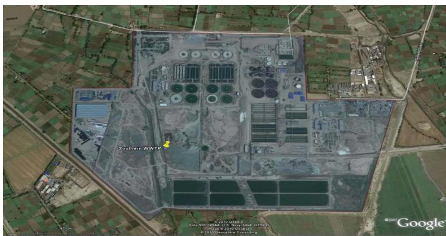
Figure 1: Tehran South Wastewater Treatment Plant facilities.
